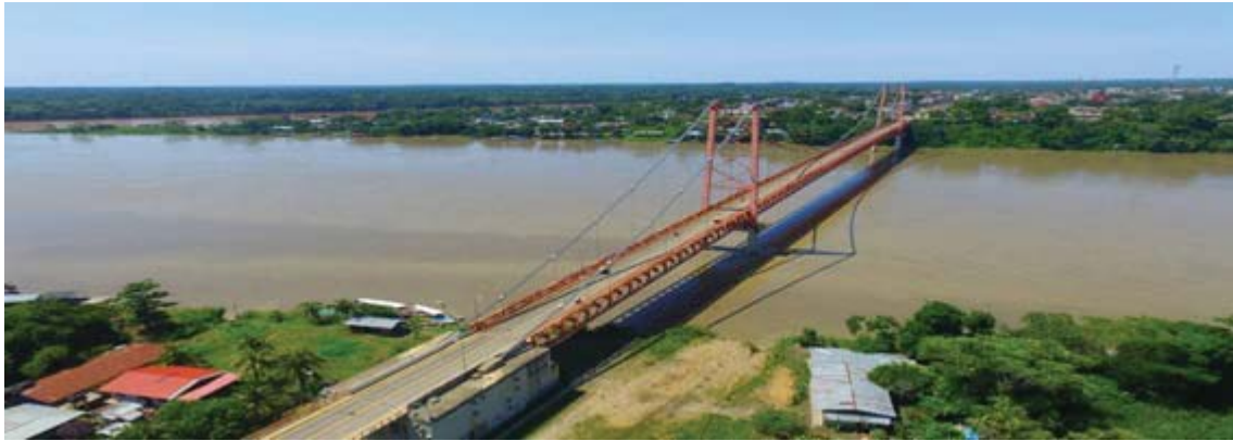
Figure 3. Billinghurst or Continental Bridge in the Madre de Dios Region. Source: IIRSA South website
