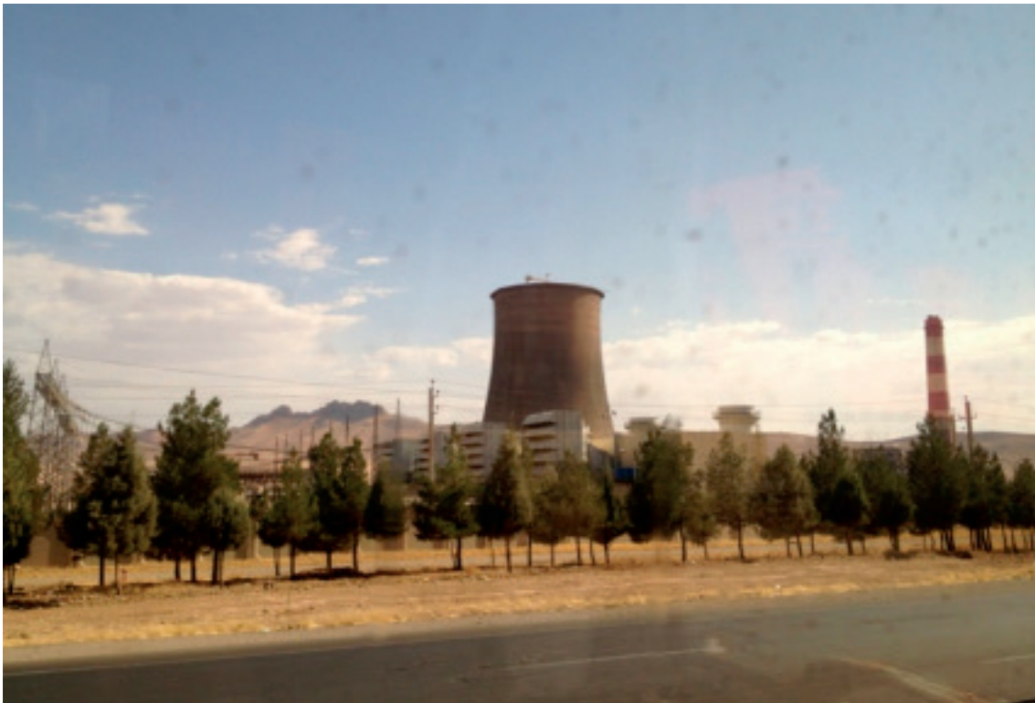
Figure 6: one of the multiple power plants in the district of Ahvaz, less than a hundred miles north to the Persian Gulf
